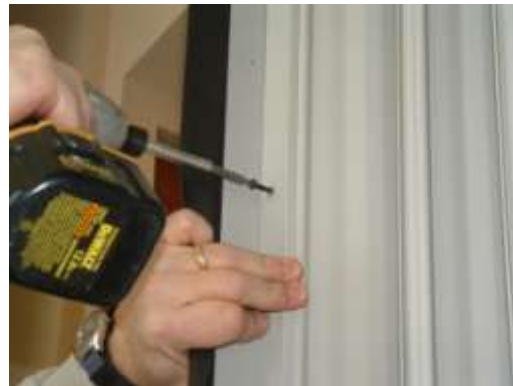
Figure 11. Attaching Jamb Section to Floating Jamb
