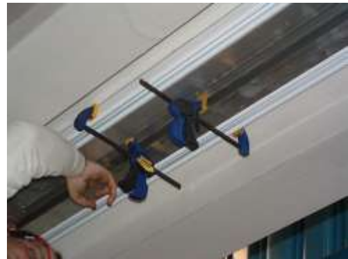
Figure 3.5.b. Using Clamps to Secure Chain
