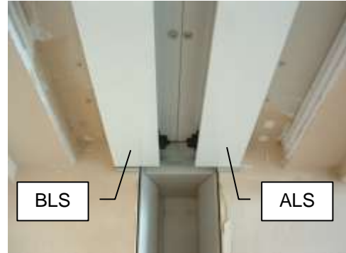
Figure 3.2. Installed Loading Section
