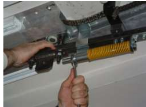
Figure 3.6. Adjusting Chain Tension
