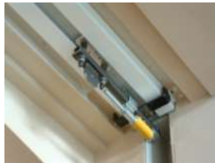
Figure 6.1. Trolley in Position for Loading Curtain
