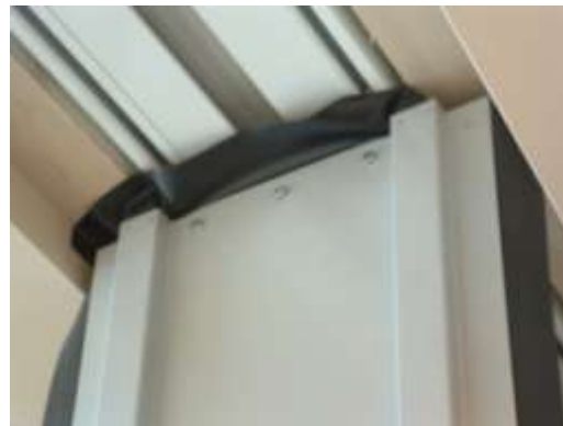
Figure 7.b. Installed Floating Jamb & Fasteners
