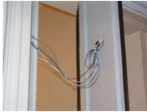
Figure 12.b. Leaving Extra Wiring
