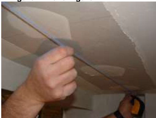
Figure III.1. Marking the Centerline
