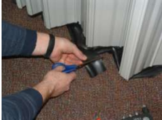
Figure 14.a. Trimming Sweep from Outside
