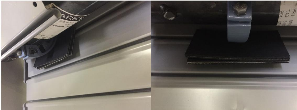
**NOTE:** The use of shims does not affect the durability or longevity of the door or any of its components.
