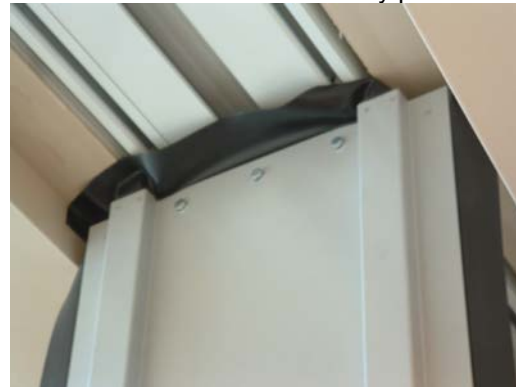
Figure 7b. Installed Floating Jamb & Fasteners
