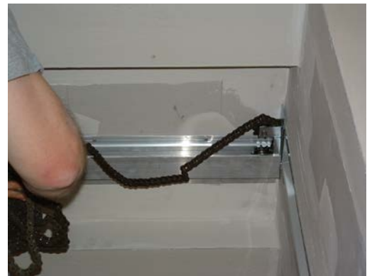
Figure 3.5a. “Threading” End Sprocket Assembly
