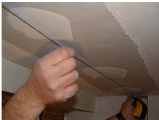
Figure III.1. Marking the Centerline
