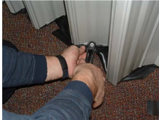
Figure 14a. Joining Sweep from Outside
