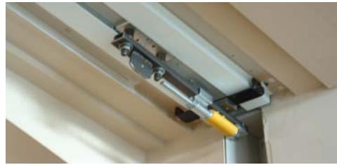
Figure 6.1. Trolley in Position for Loading Curtain
