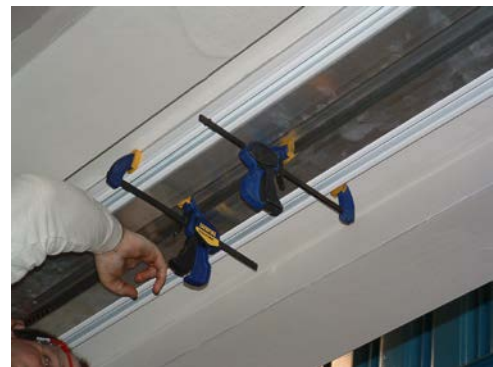
Figure 3.5b. Using Clamps to Secure Chain
