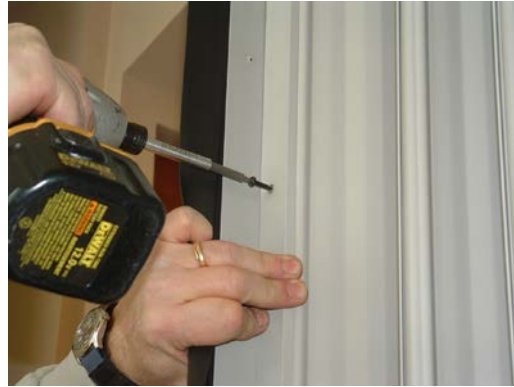
Figure 11. Attaching Jamb Section to Floating Jamb
