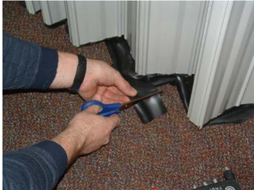
Figure 14a. Trimming Sweep from Outside
